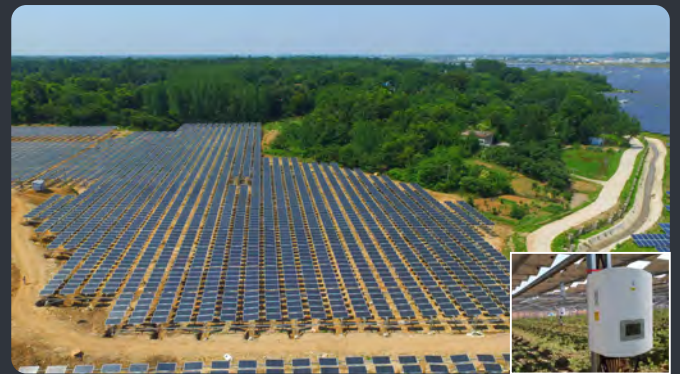
Anhui Jinzhai Agricultural-photovoltaic hybrid PV plant | 6MW
