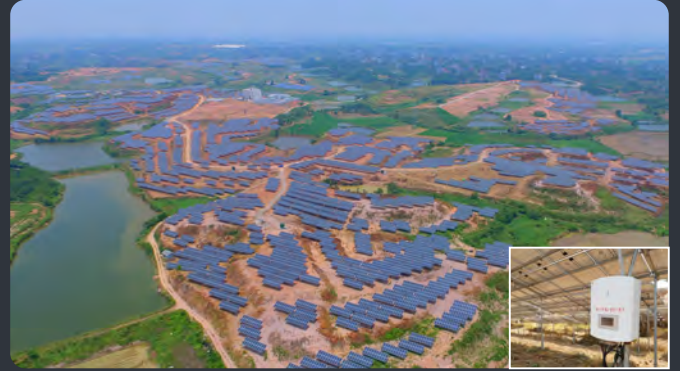
Zhejiang Longyou Agricultural-photovoltaic hybrid PV plant | 40MW
