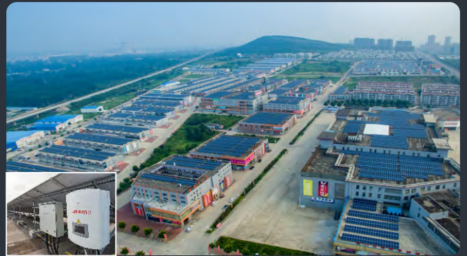
Shandong Tianqu Logistics Trade City | 5.5MW
