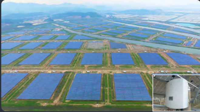
Zhejiang Shepantu Fisheries-photovoltaic hybrid PV plant | 40MW
