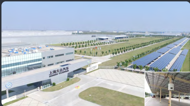
Shanghai Volkswagen Photovoltaic solar carport | 55MW
