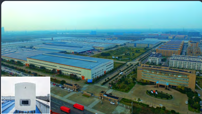
Hangzhou Bay Geely | 5.6MW
