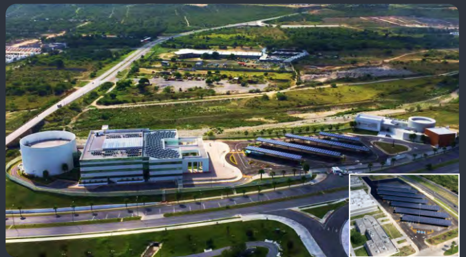
Mexico-Tamaulipas Carport | 5MW
