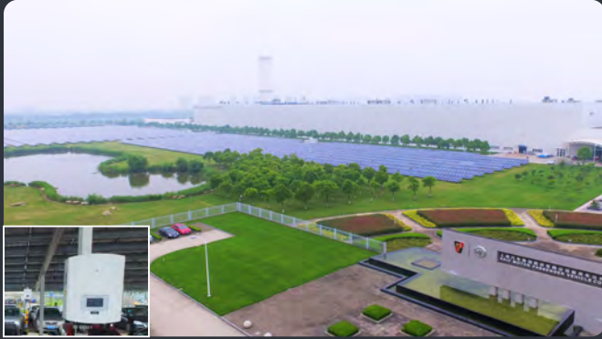
Shanghai General Motor | 5MW
