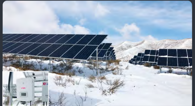
Shanxi Guangling PV plant | 1.47MW
