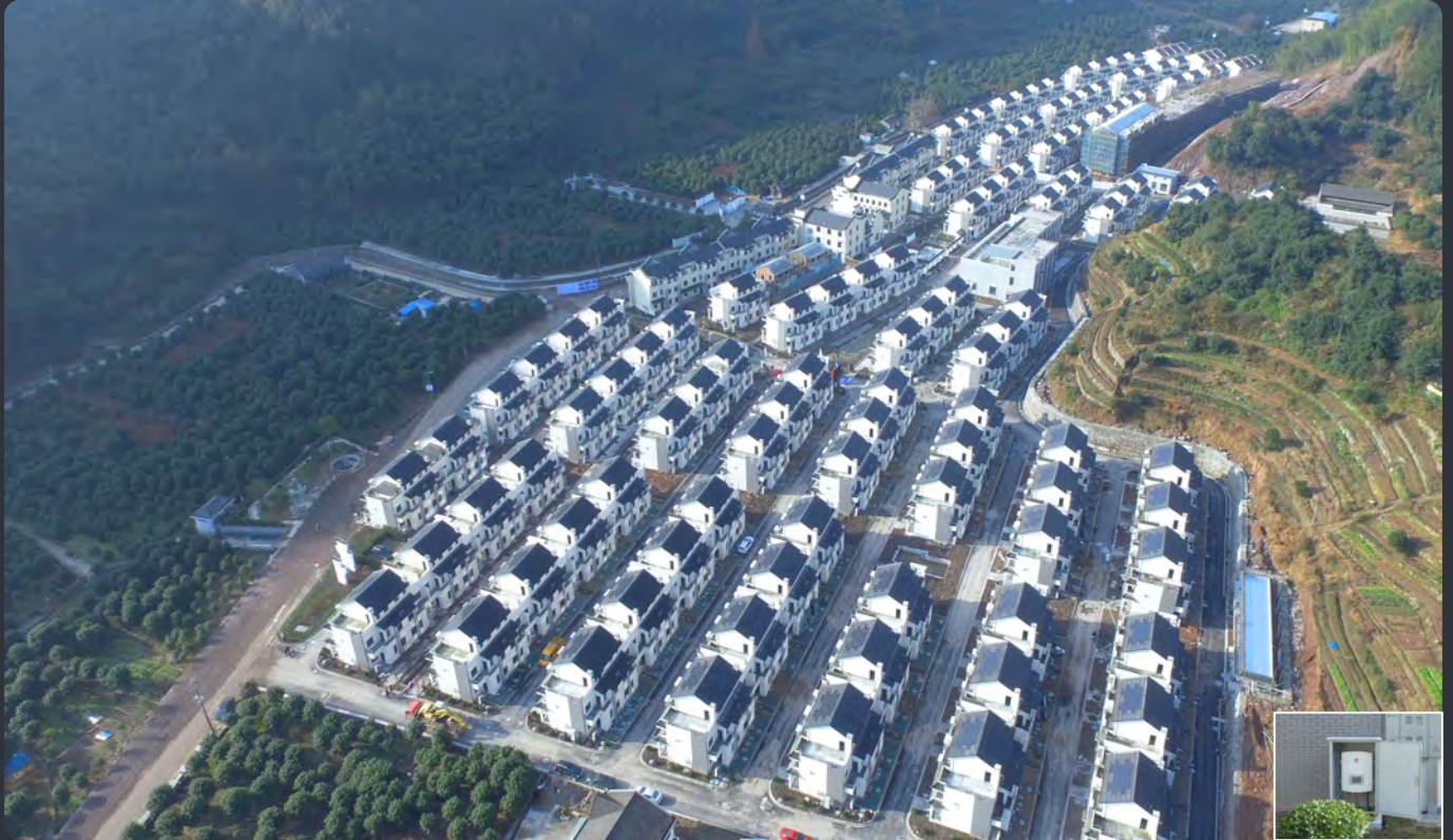
Zhejiang largest photovoltaic building integrated village | 300kW
