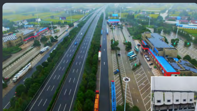
Jiaying Nanhu service area | 250kW
