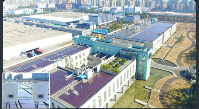
Hangzhou ABON | 410kW
