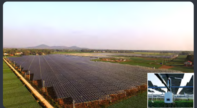
Hubei Guanyin Agricultural-photovoltaic hybrid PV plant | 20MW
